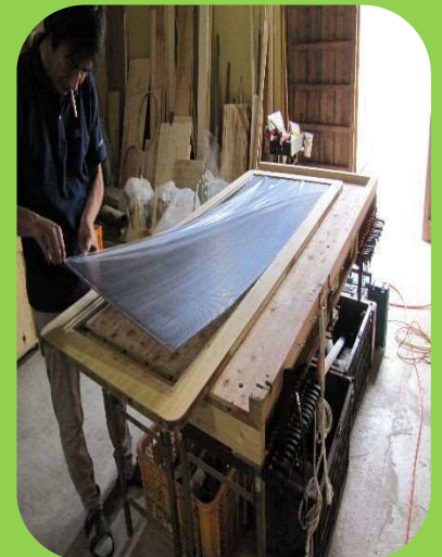
建具の組立て
